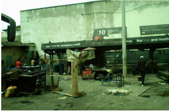
Figure: 5. 9 Dilapidated state of part of the Kenya Bus Station Terminus
