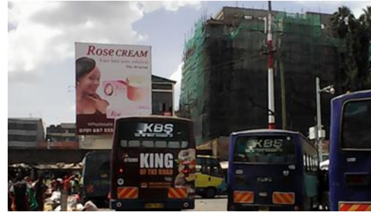
Figure: 1. 5 Upcoming development within the vicinity of the terminus Source: Author (2015)
