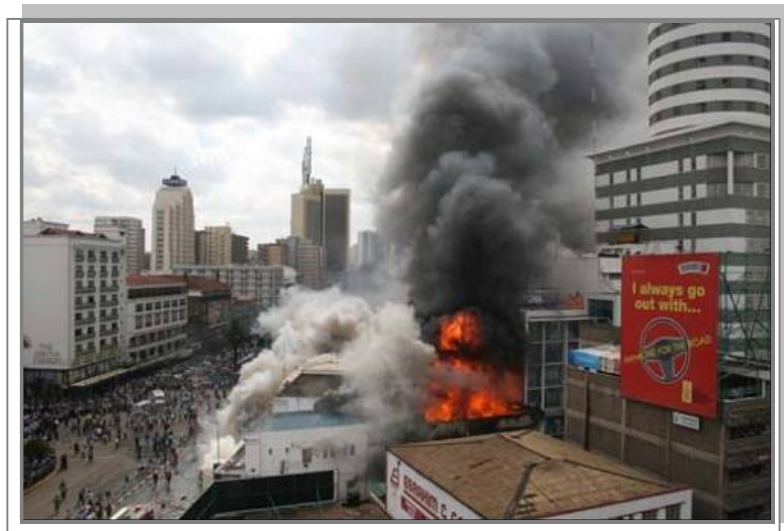
Plate 2.1: Nakumatt Downtown Supermarket fire (Source:www.irinnews.org)
