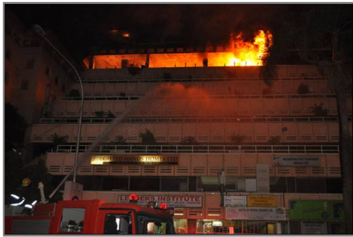
Plate 2.2: Kimathi House fire (Source: Daily Nation, online archives)
