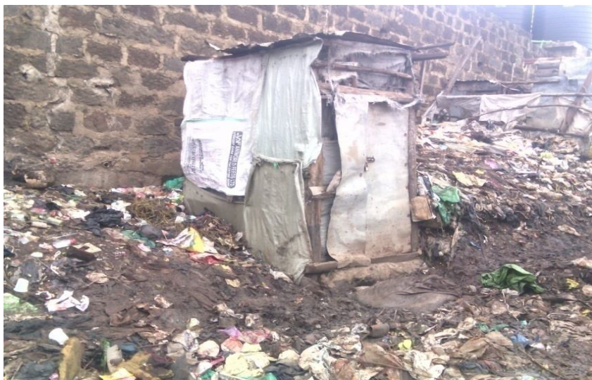
Plate 3: Simple Pit Latrine (Field Work 2015)
