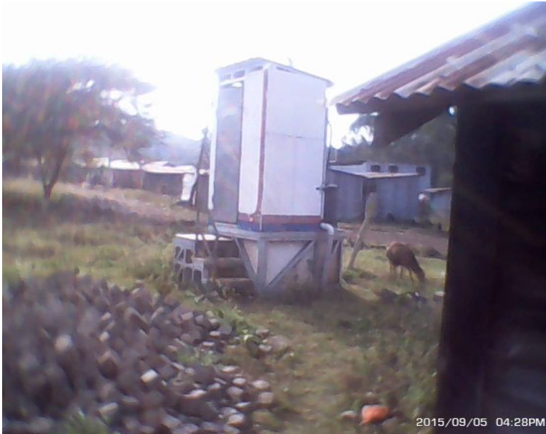
Plate 4: Skyloo Toilet (Field Work 2015)
