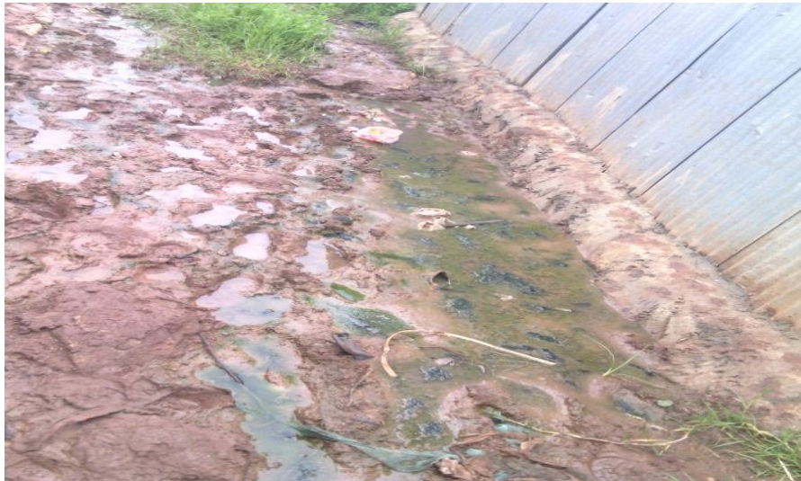
Plate 5: Water Contaminated with Toilet Overflow (Field Work 2015)
