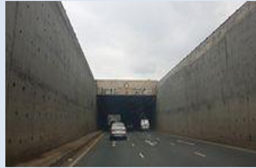
Plate 4: GSU under pass and overpass
