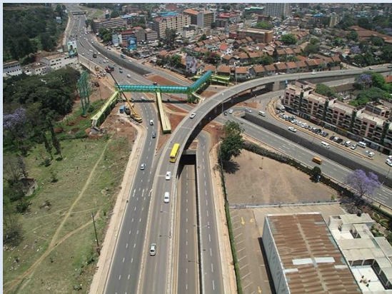
Plate 5: Forest road interchange with overpass foot bridge
