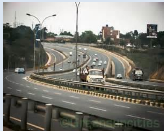
Plate 2: Upgrade to highway status of eight lanes
