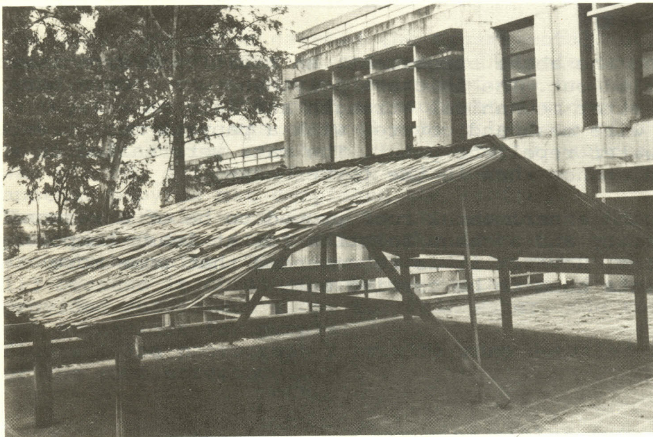
Photograph 1. Overall view of the experimental roof structure.
