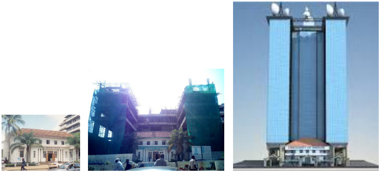
Fig. 5.19. Transformation on Oginga Odinga Street
